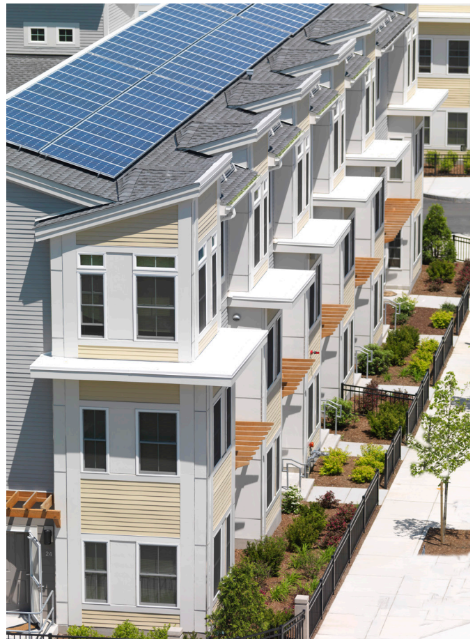
Solar panels on Old Colony BHA housing
