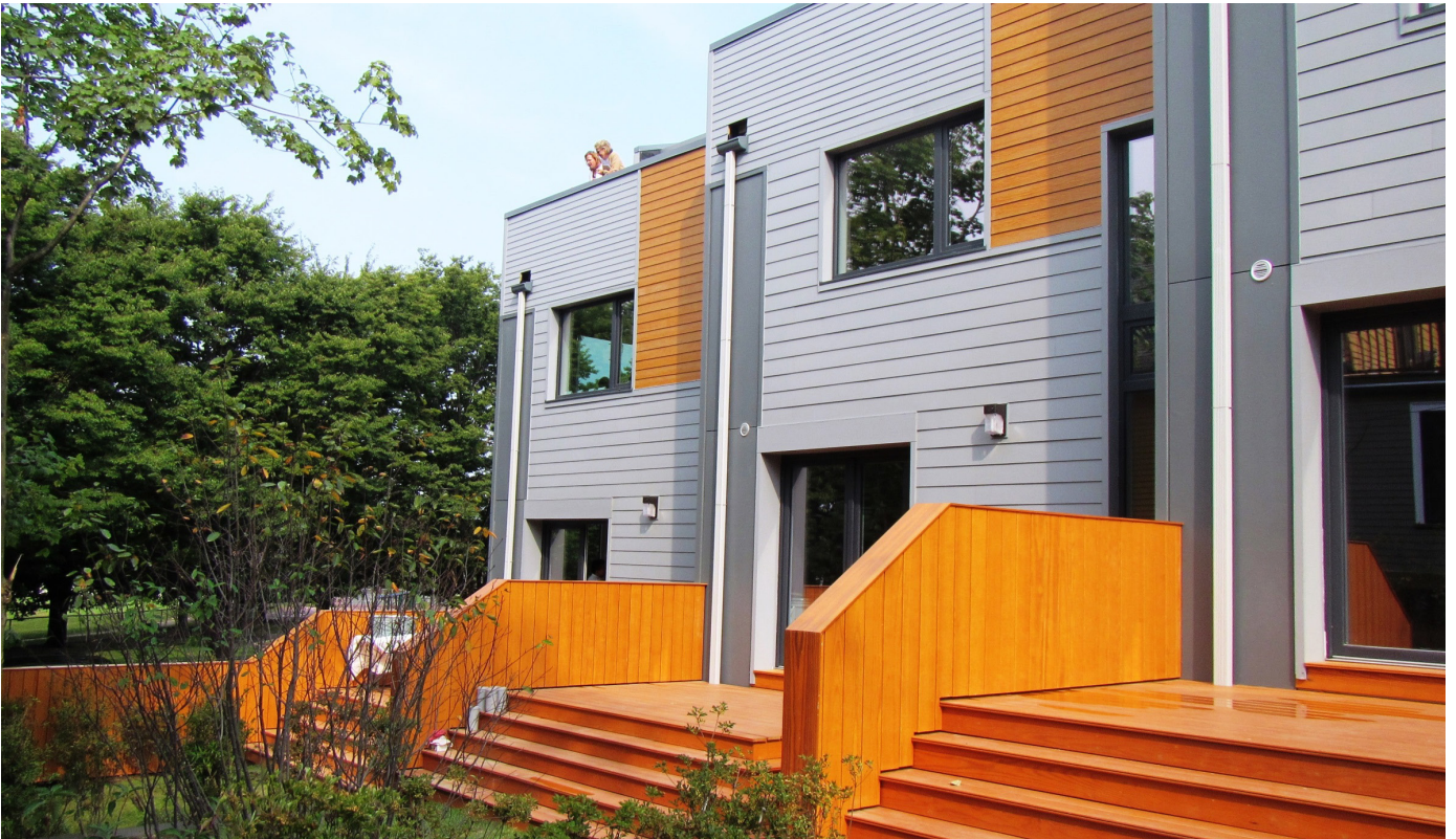
Boston's first Energy+ housing development in Roxbury produces about twice as much energy as it consumes.
